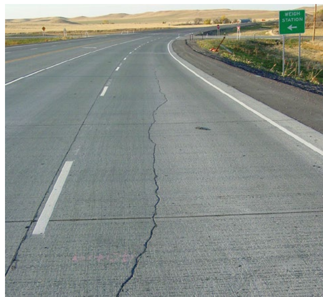
Figure 3-7. Structural longitudinal crack
