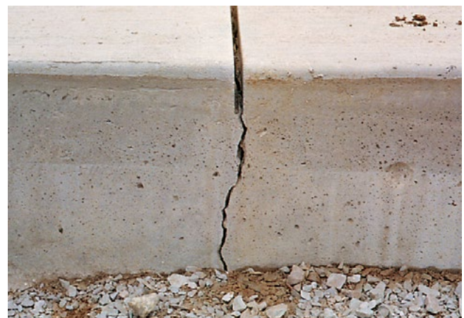
Figure 6-23. A saw cut that has cracked through as planned
