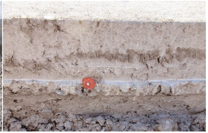
Figure 8-20. Dowel basket marked with paint for the saw crew (left) and an inserted dowel marked with a nail and washer (right)
