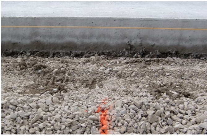
Figure 8-20. Dowel basket marked with paint for the saw crew (left) and an inserted dowel marked with a nail and washer (right)
