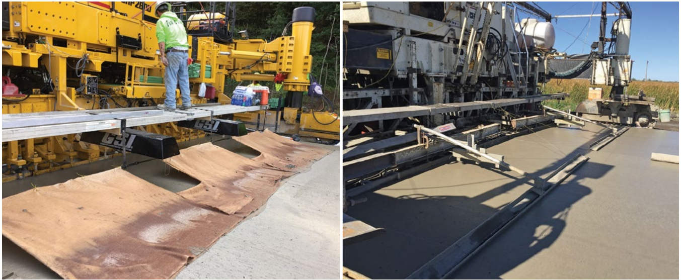
Figure 9-15. Real-time smoothness devices: Gomaco GSI (left) and Ames Engineering RTP (right)
