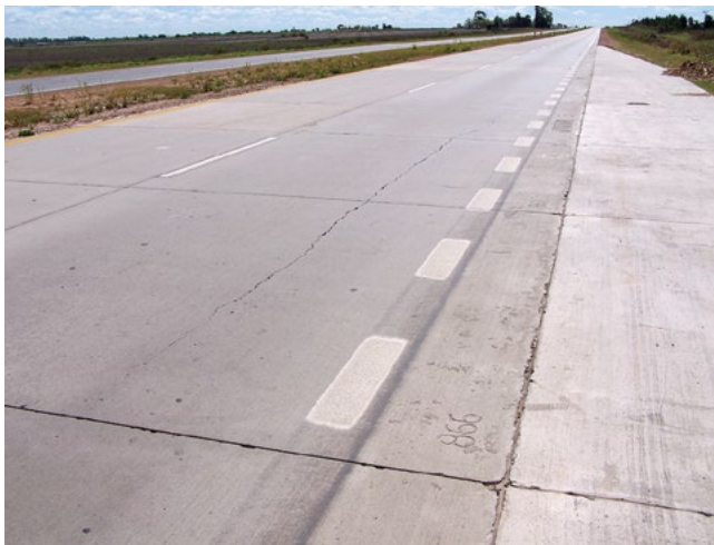
Figure 6-29. Random longitudinal crack
