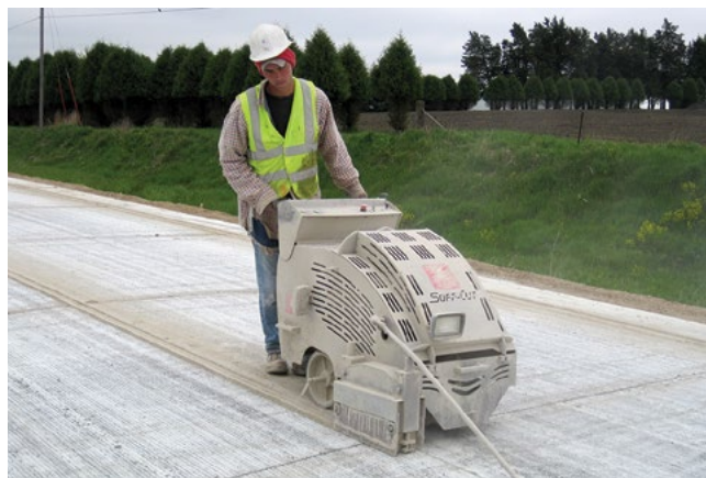
c) Early-entry, walk-behind dry saw
