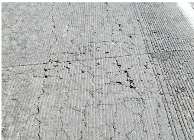
Figure 6-27. Map cracking
