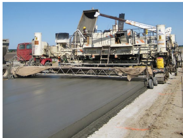
Figure 8-5. Trackline of slipform paving machine
