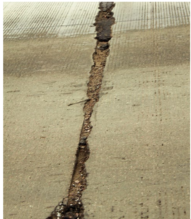
Figure 6-34. Joint damage
