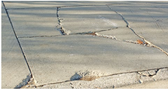
Figure 3-8. Shattered slab
